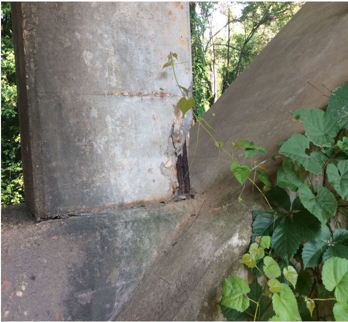
PHOTO 1 Description MINOR DELAM, CRACKING & SPALLING W / REBAR EXPOSED IN COLUMN 6 ON RT. SIDE AT END OF ARCH AT PIER 3. MINOR SECTION LOSS ON REBAR.
