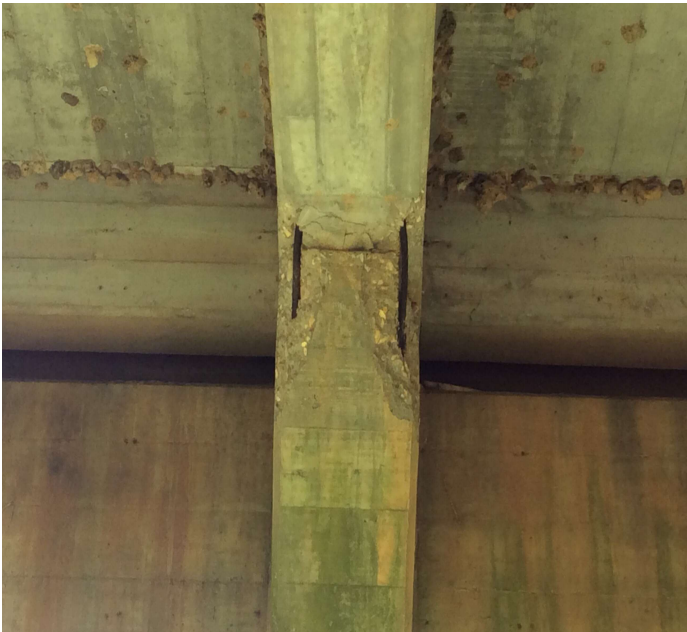
PHOTO 1 Description DELAM, CRACKING & SPALLING W / REBAR EXPOSED IN BEARING AREAS OF BEAMS.
