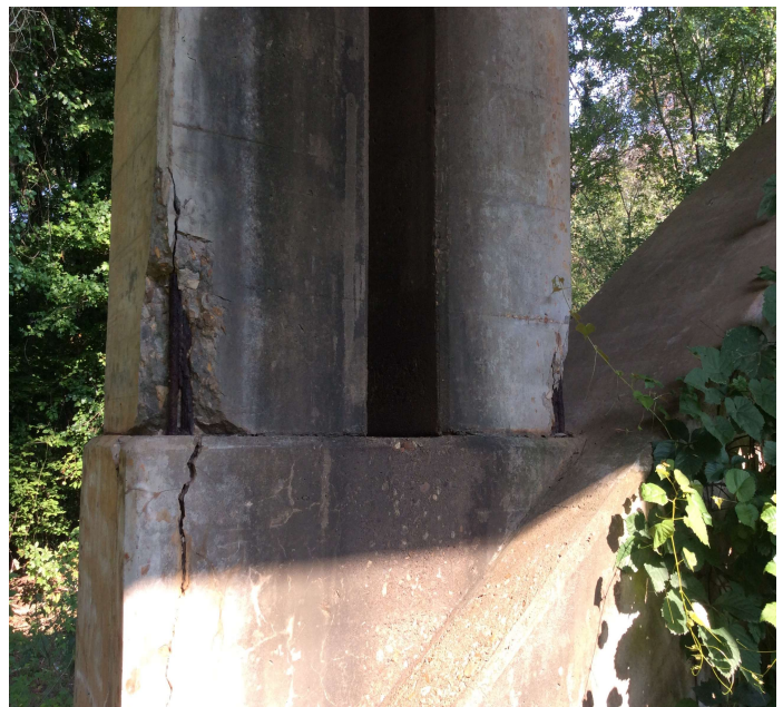
PHOTO 2 Description DELAM CRACKING And SPALLING In COLUMN 7 And PEDESTAL AT PIER 3 ON RT SIDE.
