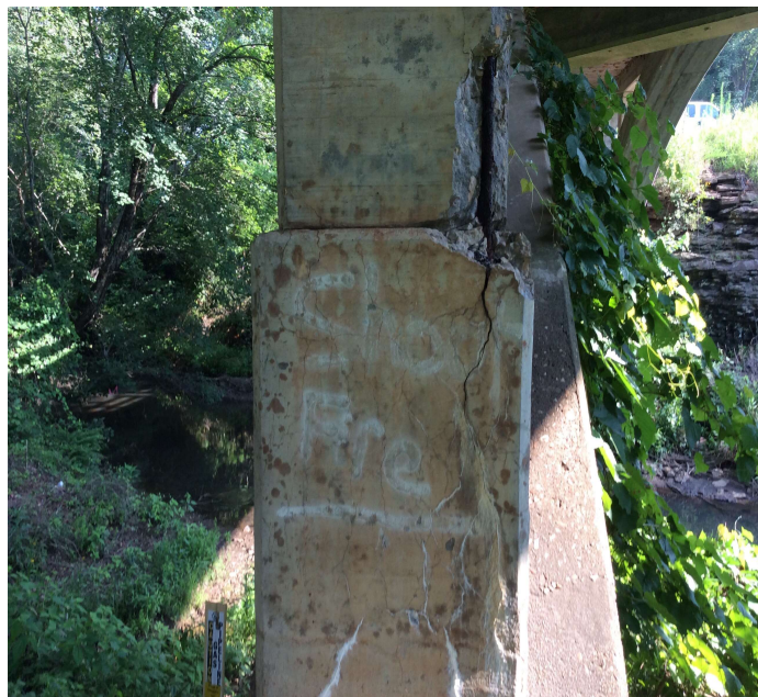
PHOTO 1 Description DELAM CRACKING And SPALLING In COLUMN 7 And PEDESTAL AT PIER 3 ON RT SIDE.
